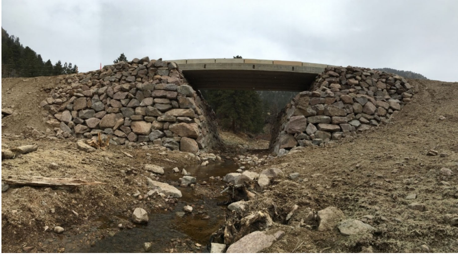
Fig. 8 Constructed GRS wall with natural rock blocks as facing
