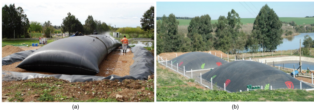
Figure 13. (a) Containment for sludge treatment, IGS photo contest 2014 (A. Teixeira), and (b) anaerobic digester lined and capped with EPDM Geomembrane, IGS photo contest 2010 (S. Murray)
