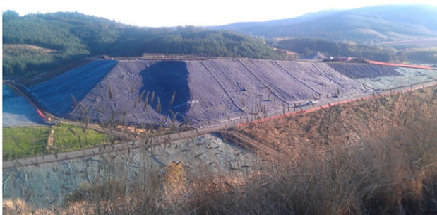
Figure 15. EPDM Geomembrane rubber temporary landfill cover used over a twenty year span, IGS photo contest 2014 (W. Johnson)
