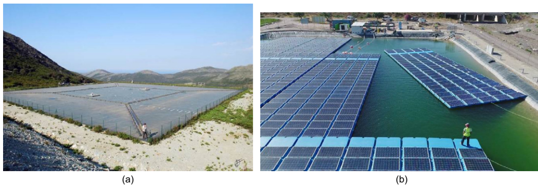
Figure 10. (a) Full Ersa (Corsica, France) reservoir (from Benedetti et al. 2009) and (b) floating photovoltaic cover (courtesy M. Redón-Santafé)
