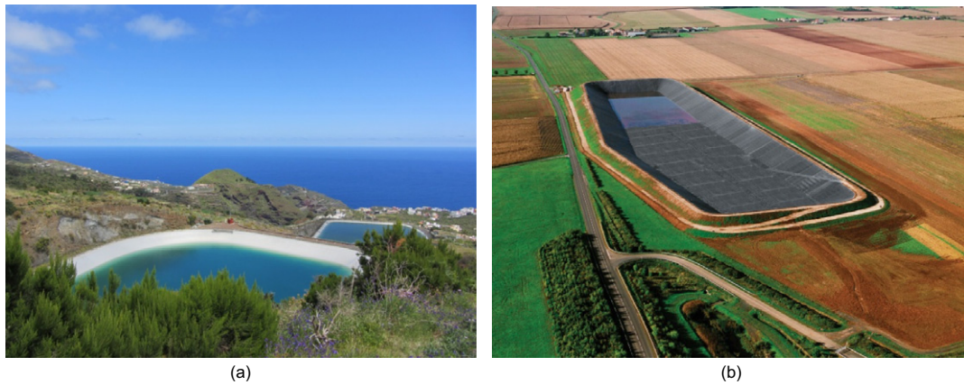
Figure 9. (a) Reservoirs waterproofed with plasticized PVC-P geomembranes reinforced with polyester synthetic fabrics (Authors: M. Blanco (CEDEX, Spain), A.M. Noval (CEDEX, Spain) & E. Aguiar (BALTEN, Spain) IGS photo contest 2014) and (b) Large irrigation reservoir lined with EPDM Geomembrane, IGS photo contest 2010 (S. Murray)
