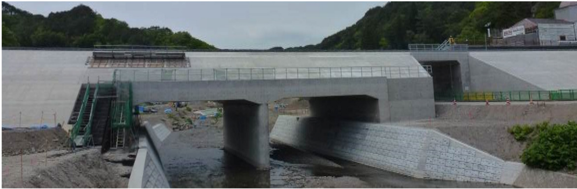
Figure 23. GRS integral bridge, Shima-no-koshi, Sanriku Railway, 20 May 2014 (courtesy F. Tatsuoka)
