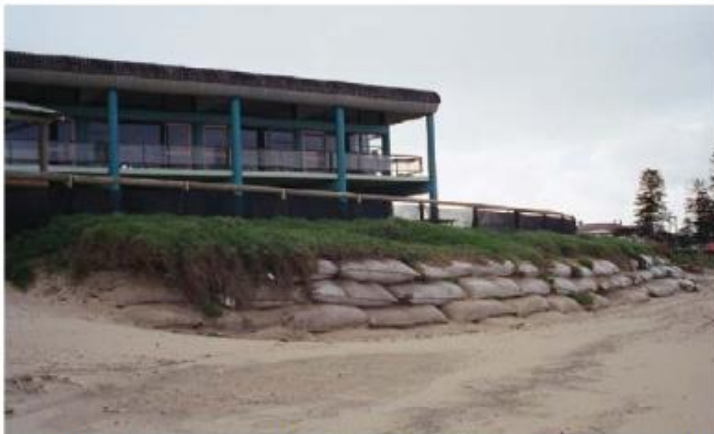
Fig. 238. Revetment made of sand-filled geotextile containers (after Saathoff et al. 2007)
