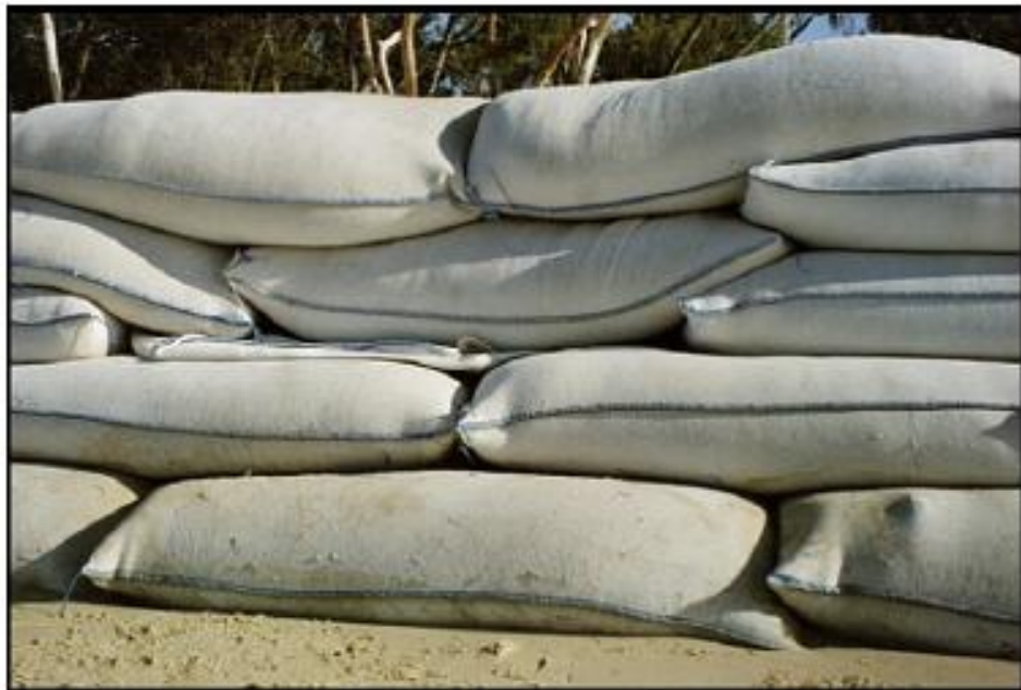
Fig. 21. Self healing characteristics of sand filled geotextile container wall
