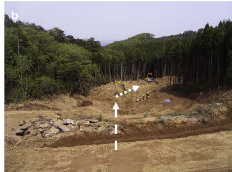
Failure of an embankment of Noto toll road (at site No. 32) caused by 2007 Noto-hanto earthquake.
