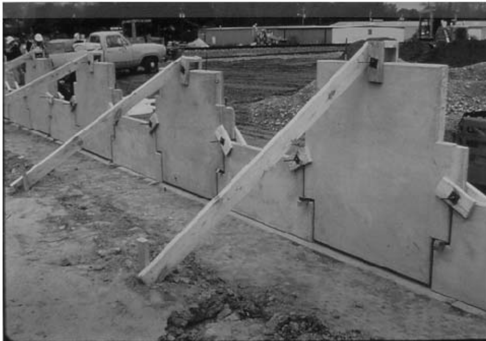
Figure 11-6. Setting first row of precast facing elements.
