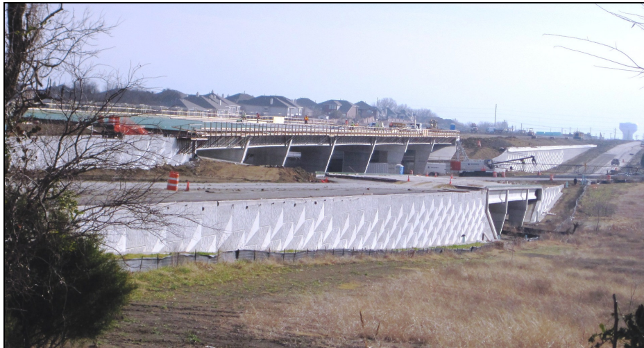
Figure 10 – Well Constructed MSE Wall
