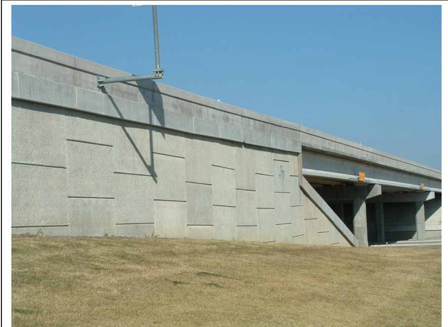
Figure 9 – Well Constructed MSE Wall
