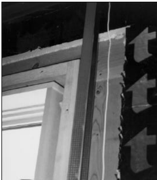
Photo 7c and 7d. Modified Window Buck at Minnesota Site
