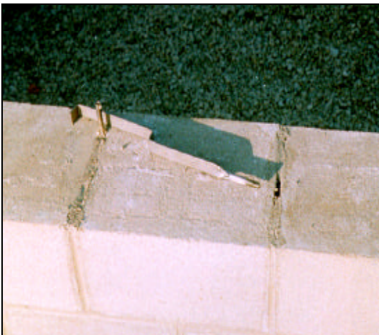
Photos 2a and 2b. Tie-Down (Anchor Bolt) at Ohio Site
