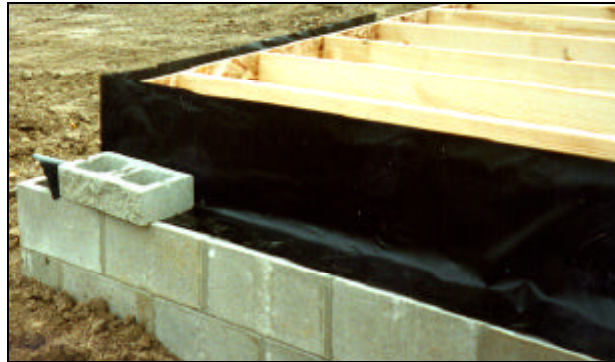
Photo 10. Moisture Barrier at Ohio Site
