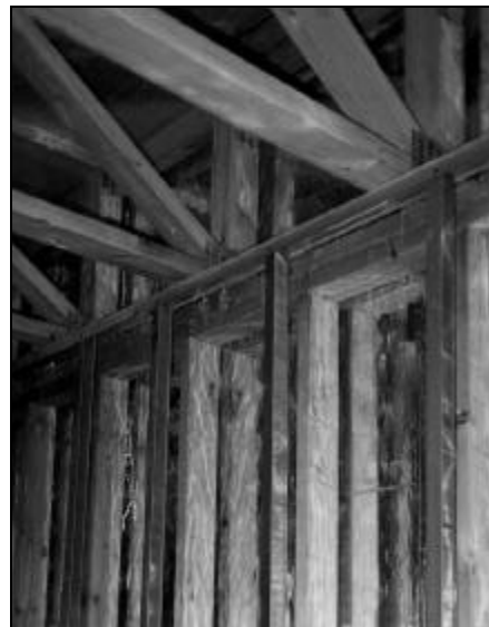
Photo 9 Floor Deck Connection at Minnesota Site
