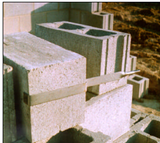
Photos 2a and 2b. Tie-Down (Anchor Bolt) at Ohio Site
