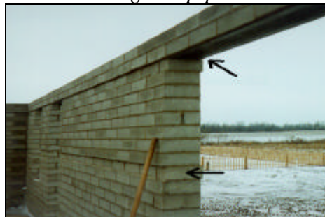
Photo 11. Channel for Drywall Nailers at Ohio Site
