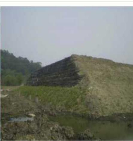
Fig. 1. The RSW on soft clay.
